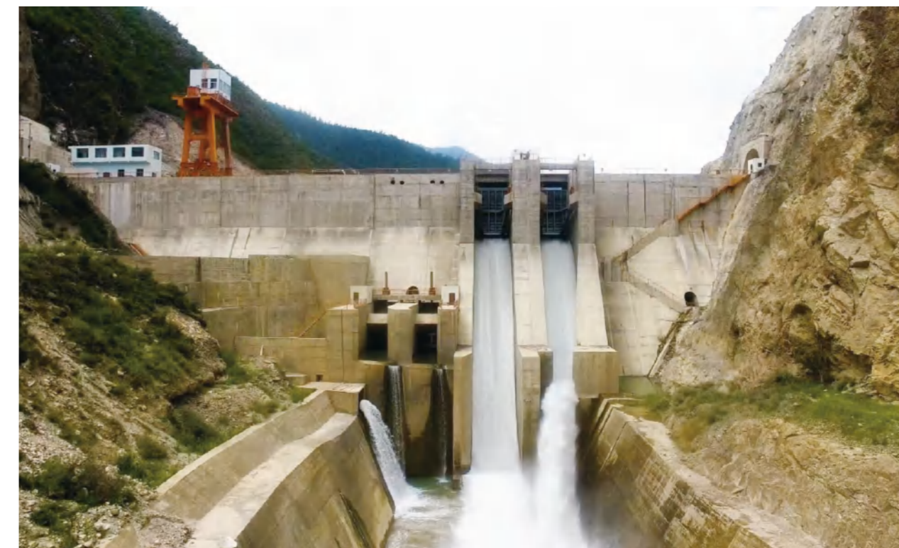
九龙峡水电站大坝工程 Jiulongxia Hydropower Station dam project
